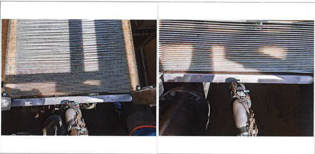
MB 2, Unit 3 broken top clip trimmed
