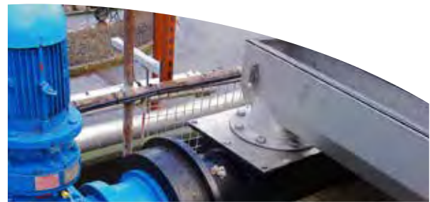
Flanged opening to accommodate existing launder channel.
