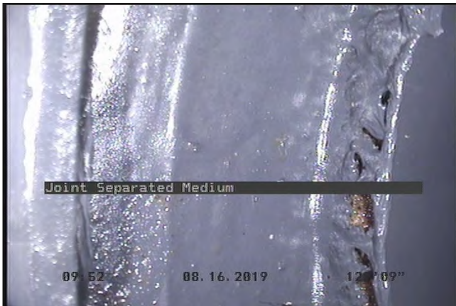
Photo: 50-19-JSM-11.JPG 129.74FT, Joint Separated Medium
